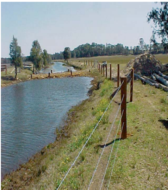
Fencing off drains from stock is a remediation option being implemented in the Clybucca and Tuckean Swamp as part of the Environmental Services Scheme.
