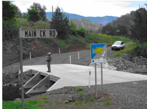
Same road crossing designed to allow fish passage
