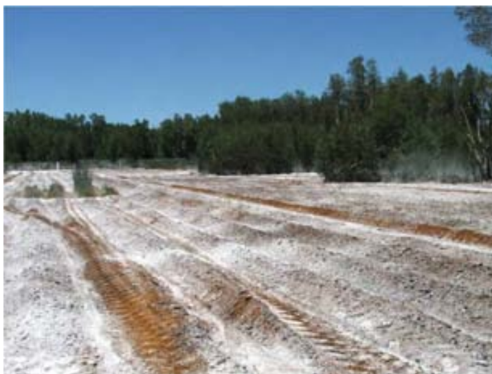
Site preparation – ridged & furrowed with lime applied
