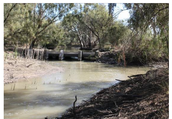
The current structure viewed from upstream. The structure was partially remediated by taking out the drop boards and removing a sill that created a 20cm drop (native fish are hindered by a drop of as little as 10cm). Further remediation is now being undertaken to reduce the velocity of flow, which has also been identified as hindering the passage of native fish at this site. Photo: Rodney Price.
