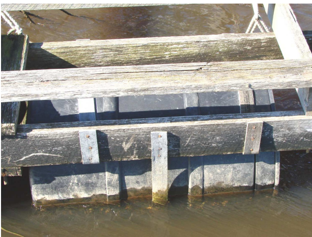
Figure 10. A 200 litre plastic drum secured to longitudinal raft timbers by two cushioning top shoulder straps and a drum girth strap.
