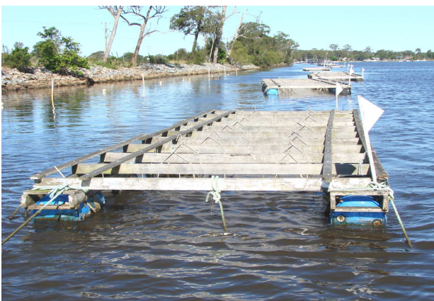
Figure 1. A Typical drum raft constructed using recycled 200 litre plastic drums.
