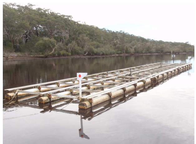
Figure 3. A Typical pipe raft constructed using large diameter (300mm) PVC end-capped plastic pipe.
