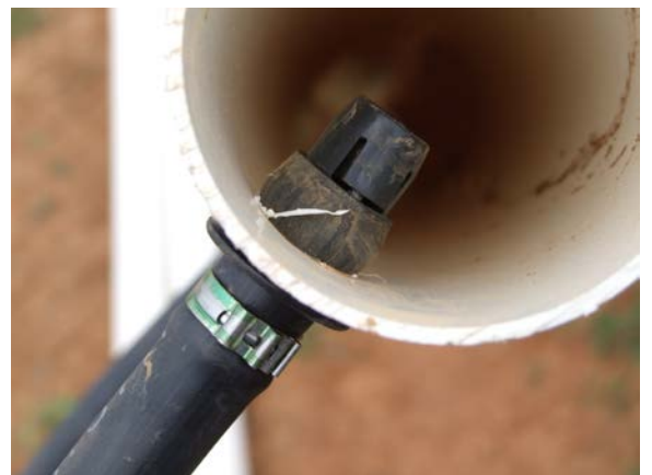
Drip tape connected to the PVC pipe. Image: S. Priest
