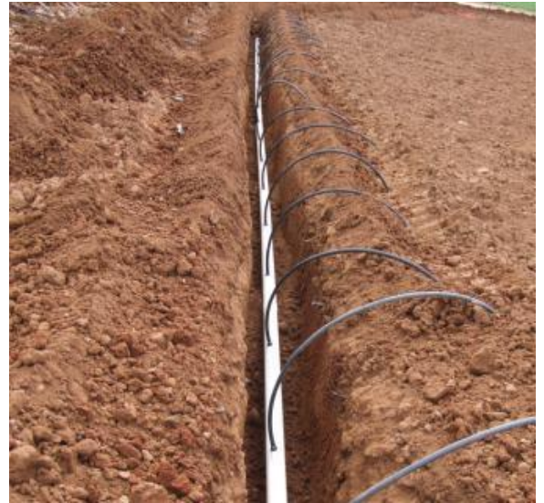
Sub-mains in the trench. Image: S. Priest
