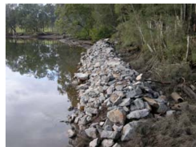
Rock fillets protect young mangroves against wave action erosion. Photo: I&I NSW
