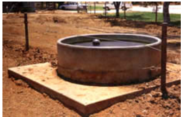
Figure 3. Round trough in fence line
