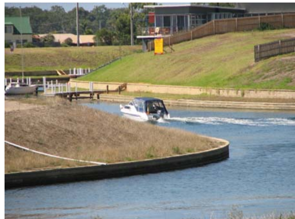
A new canal estate at Paynesville.
