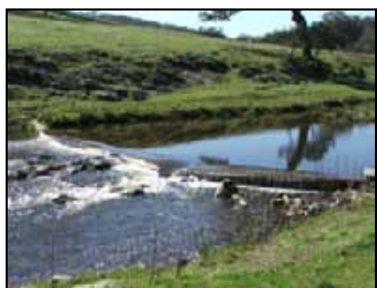
Plate 6: Water gauge structure, Cockburn River, Tamworth LGA (Code: WGS13).
