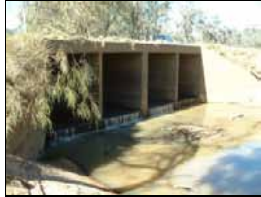
Plate 2: Box culvert, Gunidgera Creek Narrabri LGA (Code: UPN6).
