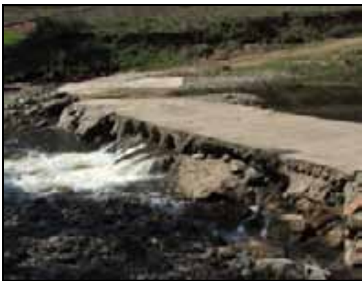
Plate 25: Swamp Oak Creek Culvert (CR37)
