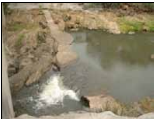
Plate 16: Concrete Capped Pipe (LPRB)
