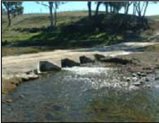
Plate 29: "Plumthorpe" Culvert (UMA73)
