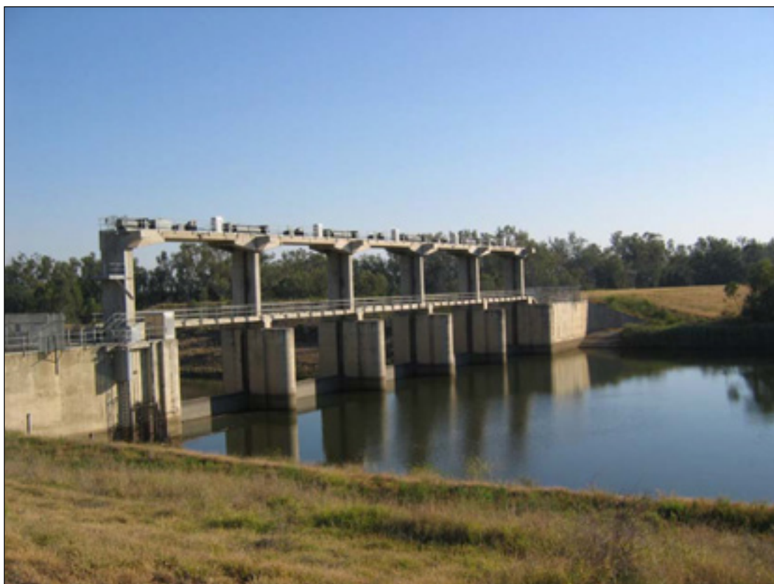
Figure 1. Boggabilla Weir, Macintyre River view from upstream side on the left bank (369.317ML/day).
