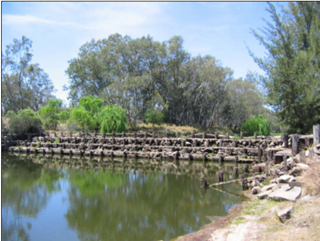
Figure 1. Cunningham Weir, Dumaresq River view from the left bank (0 ML/day).
