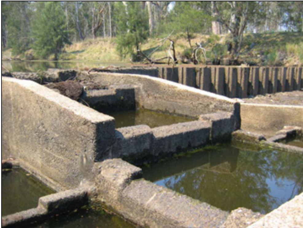
Figure 2. Pool-type fishway, Glenarbon Weir.
