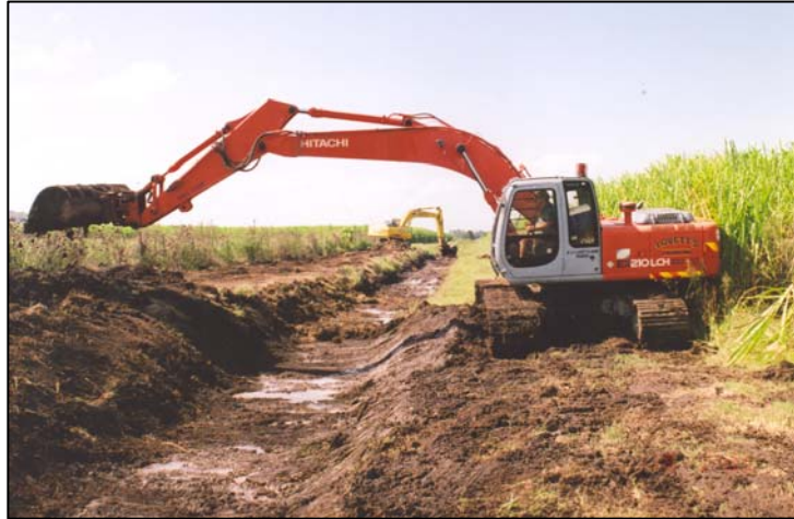
Reshaping drains so they are wider and shallower.
