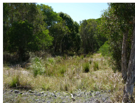
A site where a rock baffle (foreground) has been used to slow stormwater through a vegetated retention basin, enabling greater capture of sediment and nutrients and enhanced infiltration to groundwater. Photo I&I NSW
