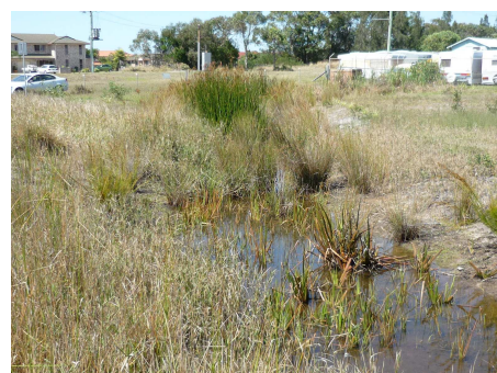
A grassy swale associated with a natural drainage line helps reduce the amount and velocity of water exiting a light industrial area. Photo I&I NSW
