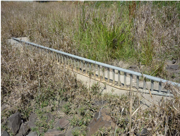
An example of a 'trash trap' downstream of a reed bed into which stormwater flows. Photo: I&I NSW
