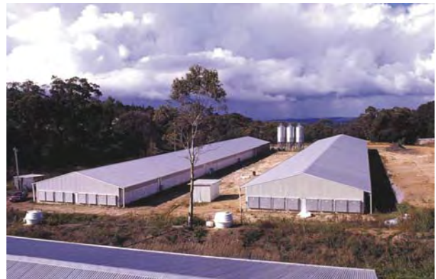
Figure 2, Sheds located in an isolated site. Photo: G. Johnston
