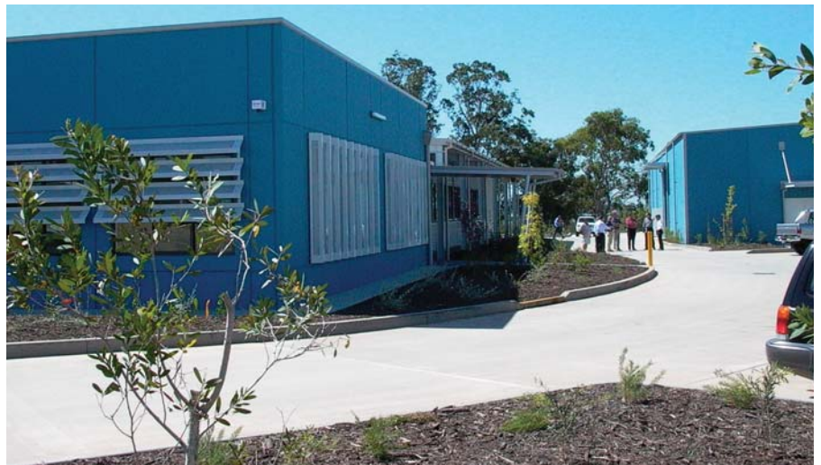
Mine Safety Technical Services in Hartley St Thornton, on the outskirts of Maitland
