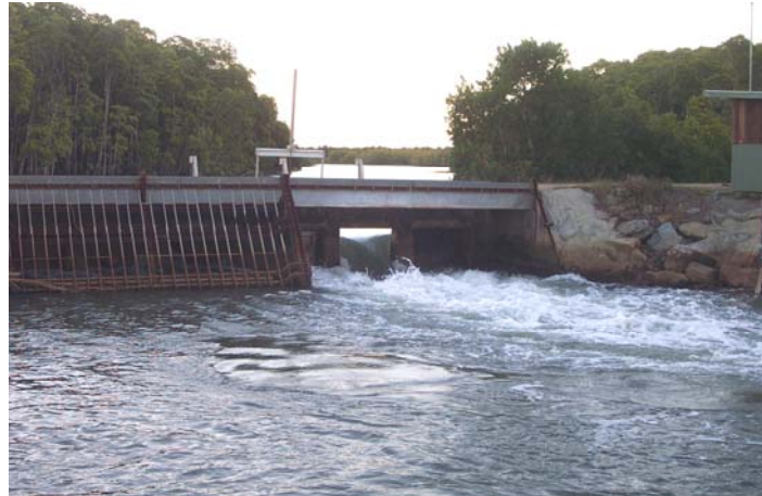
Tidal flow restored through Hills Creek floodgates.
