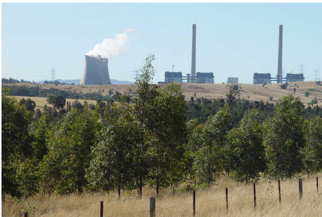
Soil amendment trial ( Corymbia maculata ): Bayswater Power Station
