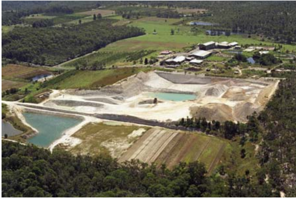
Maroota Sandstone Quarry, progressive rehabilitation in foreground. D Barnes
