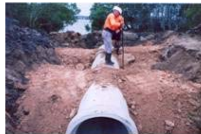
Contractors laying the new floodgate pipe. Photo: F.Welsh
