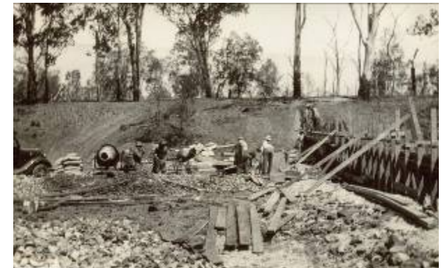
The construction of Reilly's Weir. The recent installation of a fishway on this structure is giving fish access to habitat that have not had since 1936.
