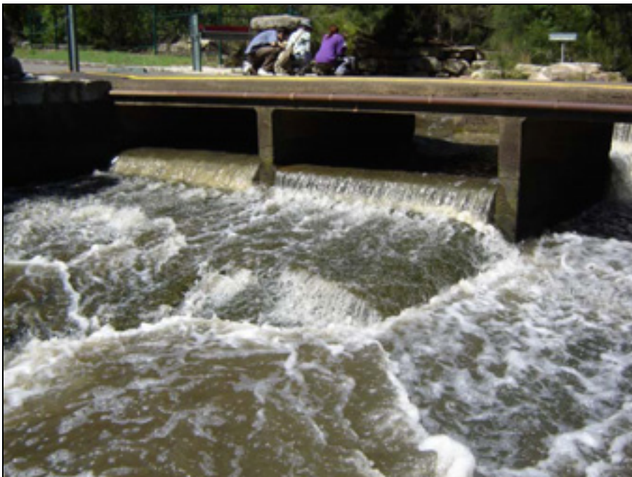
Figure 2. Entrance to fishway at moderate river flow showing headloss, flow depth and slope gradient at low tide (3/2/2005).
