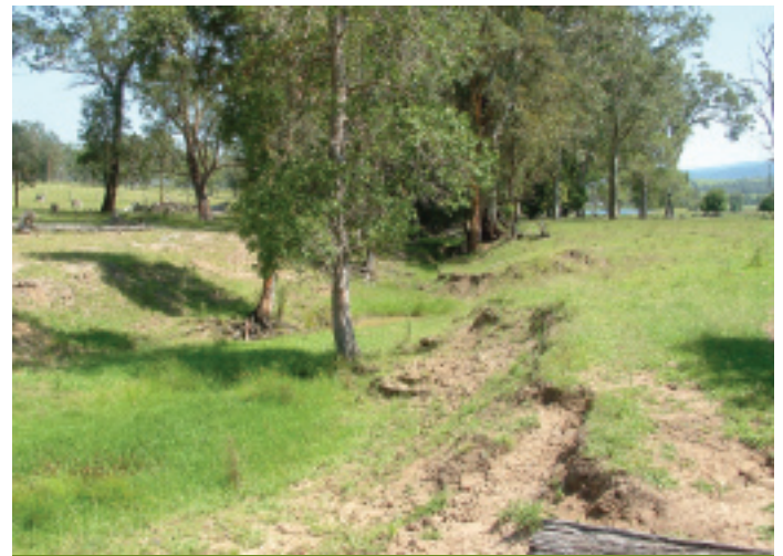
Erosion in the gully
