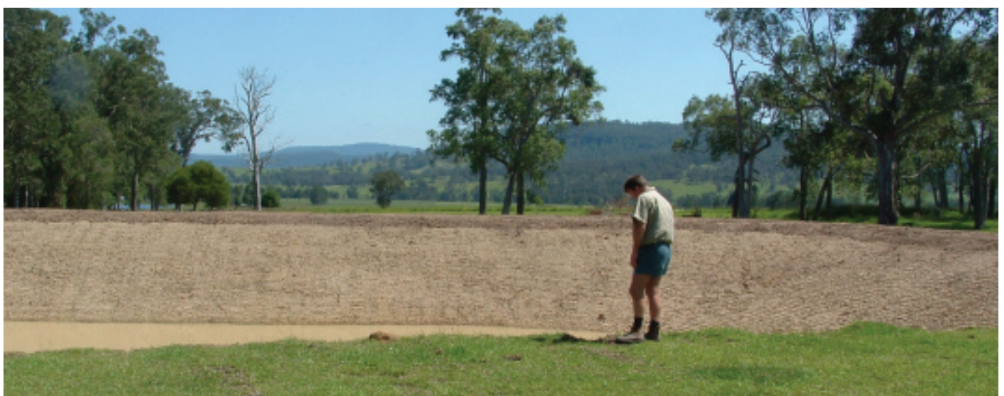
Kevin Coonan inspects the new dam
