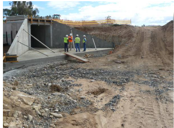
New boxed culvert tunnel under construction
