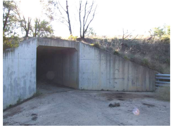
Tunnel positioned on the diagonal relative to roadway
