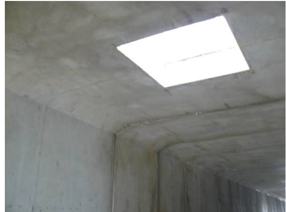
Skylight producing direct light – this light should be diffused to stop animals baulking at shadows
