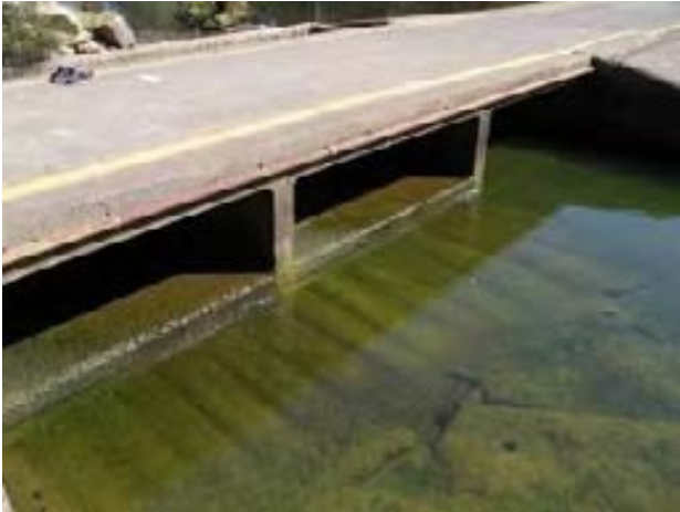
Above: The original culverts at low tide, and the new fishway near high tide. Photos: Scott Nichols NSW DPI
