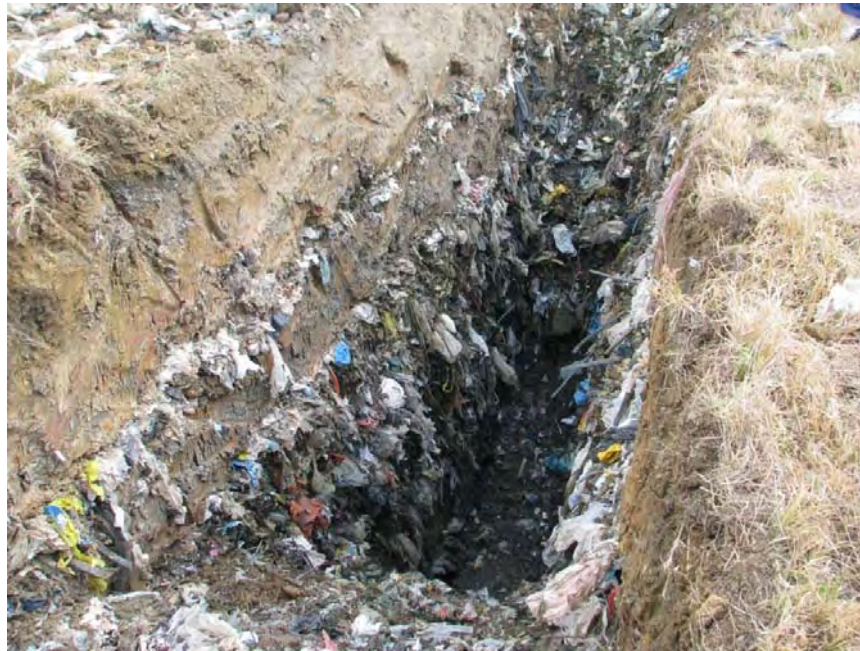
Eastern Creek landfill excavation. Photograph by Fabiano Ximenes.
