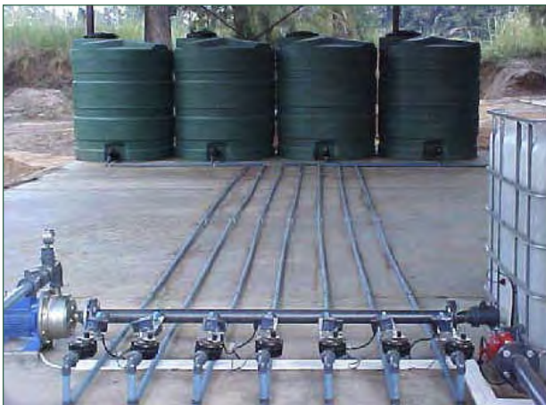
Figure 2. Multiple mixing tanks allow the supply of different fertilisers in the one irrigation shift.
