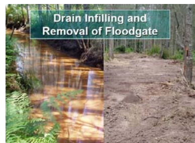
Before and after drain infilling. Photo: GLC
