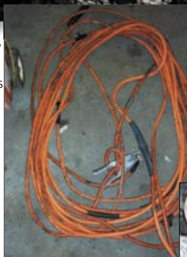
Welding practices need improvement
