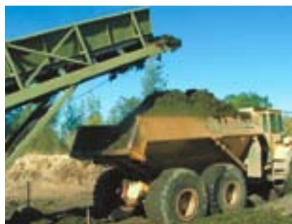
Unloading from shore conveyor into a dump truck.
