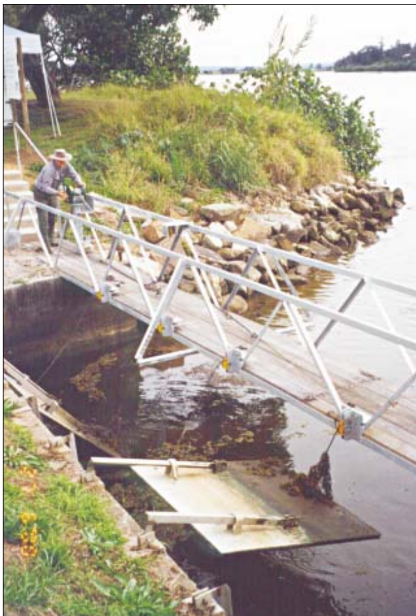
Figure 53: Opening up floodgates using a horizontal winch system on a drain in the Clarence River. Floodgate opening devices and opening strategies should be tailored to suit management objectives and the characteristics of individual drainage systems. (Photo: Alan Cibilic)
