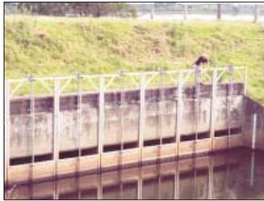
Figure 42. A large set of penstocks in a drain on the Clarence River floodplain. This set is located near the river levee on the floodgate headworks. Penstocks can be used to retain water in the drain. (Photo: Rob Lloyd)
