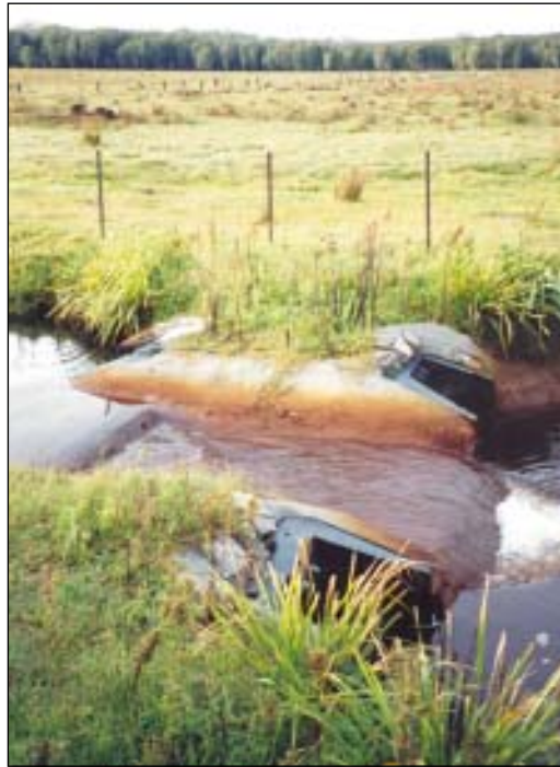
Figure 44. Weirs provide more permanent water retention. This one is used to maintain high drain water levels and reduce acid groundwater seepage.
