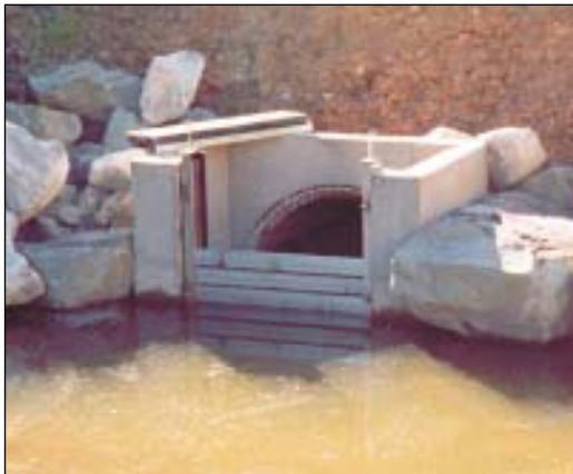
Figure 43. dropboard culverts are a simple way to retain water to a desired level. Leaving a space between the boards and the pipes helps provide better drainage of overtopping waters. (Photo: Rob Lloyd)
