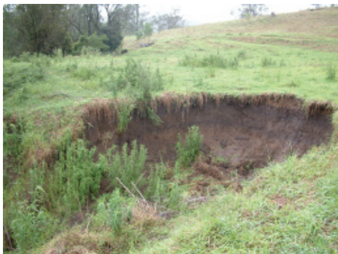
The gully head before works
