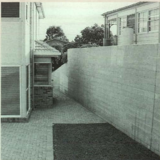
Example of extreme excavation (cut) for concrete slab
