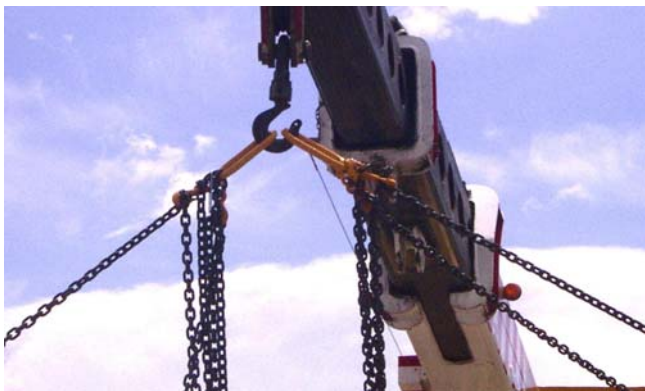
Photo 1 : Load with wide angle of separation of lifting chains
