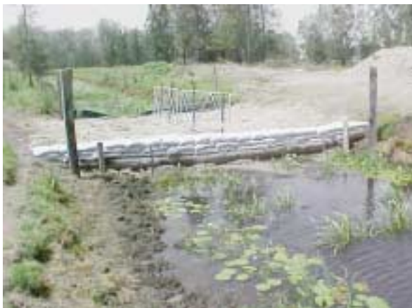
One of the weirs recently installed on the Macleay Floodplain.
