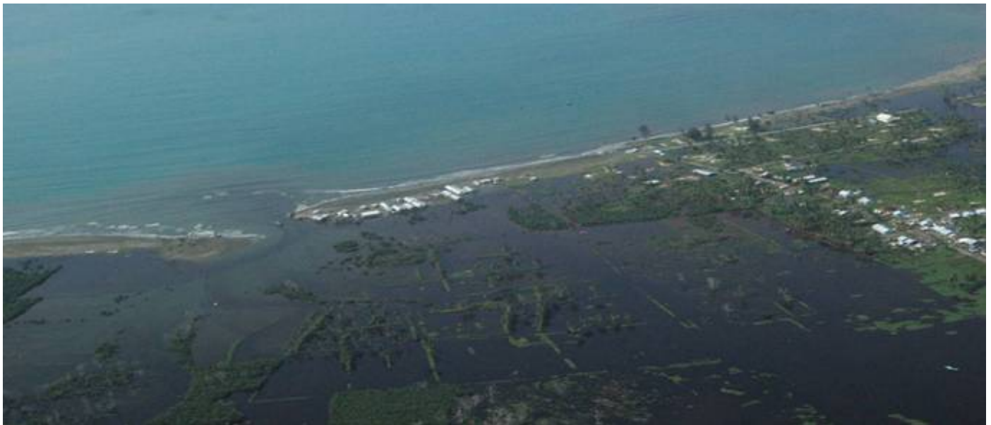
Earthquake and tsunami damage have drastically altered the hydrology of parts of the western coast of Aceh.
