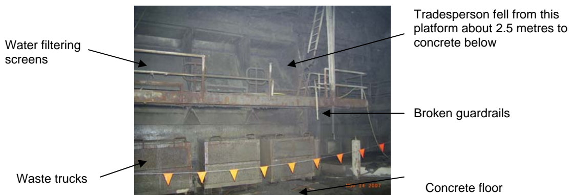
Photograph of fixed underground plant
