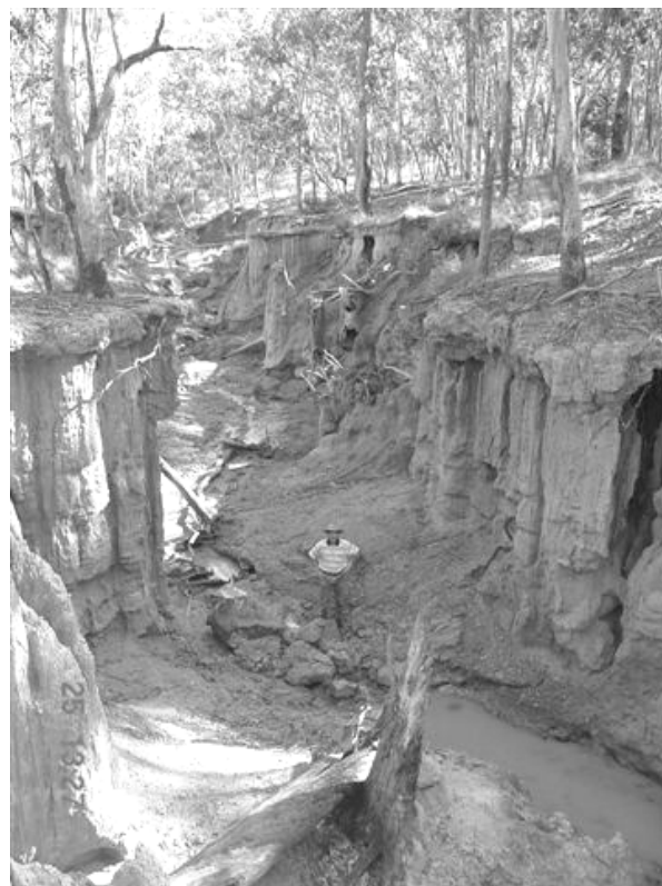
Below: Severe gully erosion in the Upper Mann catchment, photo courtesy P Roberts
