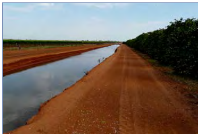
Figure 13. The 1.2 km storage channel constructed to collect and recycle irrigation water on Vince's farm.
