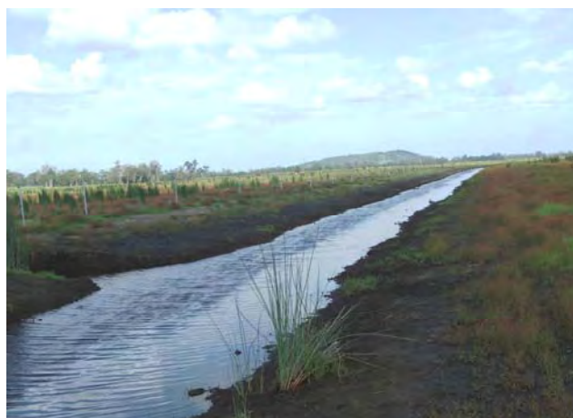
Haughwoods Canal remodelling completed, with fencing for stock control.
