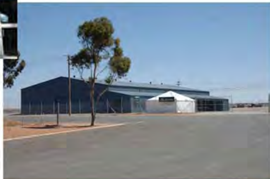
EC Andrews Regional Core Storage Facility, Broken Hill
