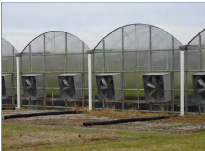
New greenhouse development and rolling bench system at Philip Ruck's nursery.
