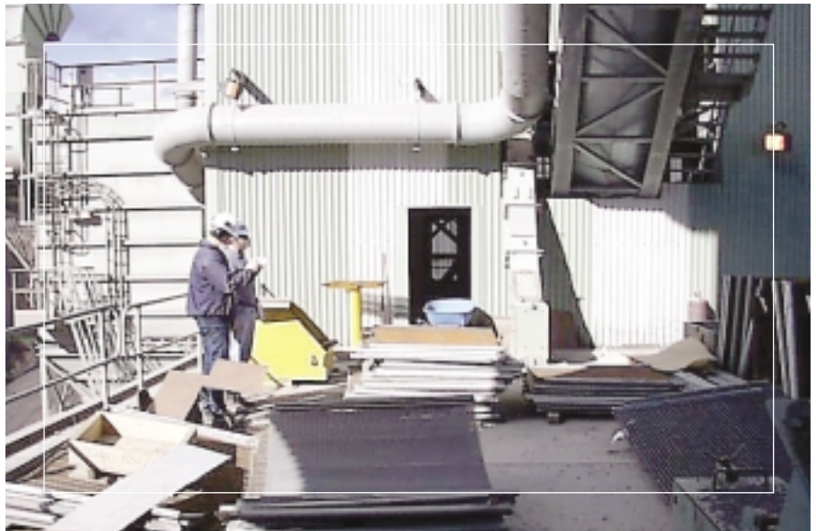
On site assessment of access walkways.
