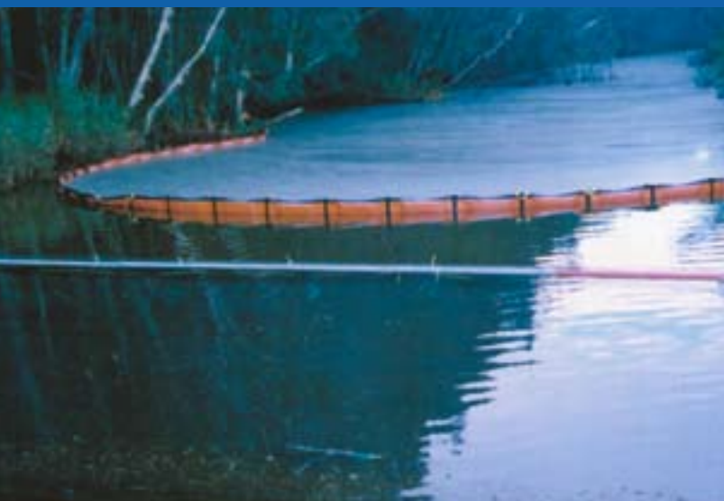
Fine mesh containment fence on the downstream side of the boom.
