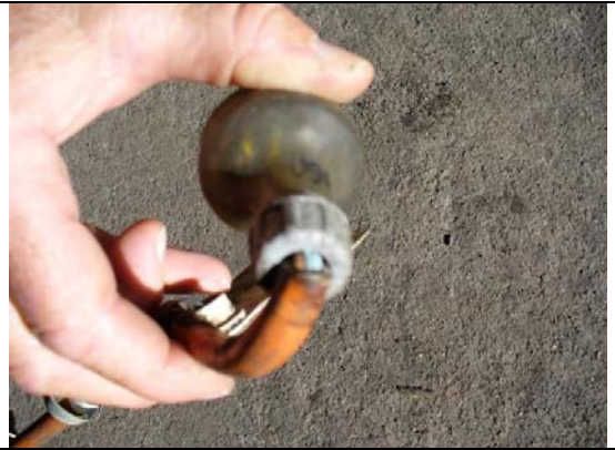
Defective cable connection to the plug
