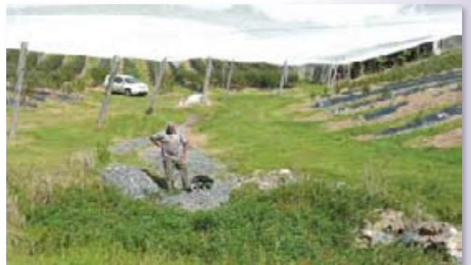
Fig 12: Subsurface pipes in the orchard 12 months after completion covered with groundcovers
