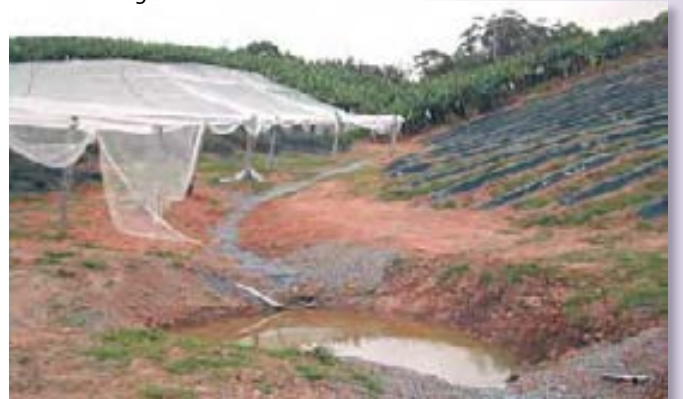
Figure 13: Subsurface agricultural pipes laid below the surface keep springs below the ground level in an orchard
