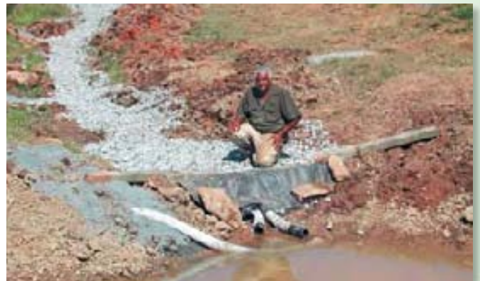
Figure 6: Sub soil drains were installed to flow into sedimentation pond
