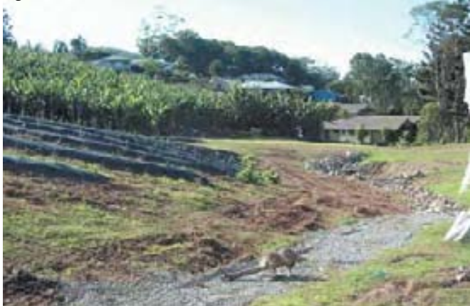
Figures 10 and 11: Agricultural pipes laid underground and covered with gravel
