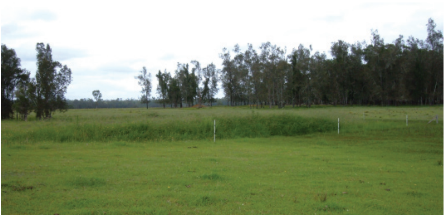
The diversion bank seen from upslope
