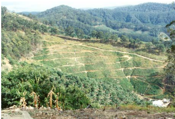
A banana plantation with correctly constructed roads running across slope.
