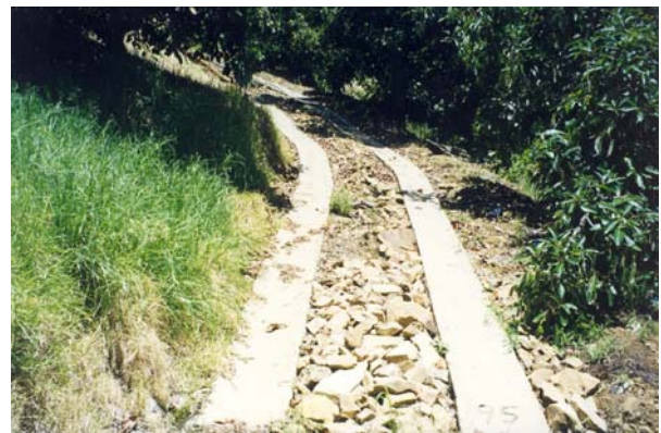
Concrete tracks may be required for steep or problem areas.
