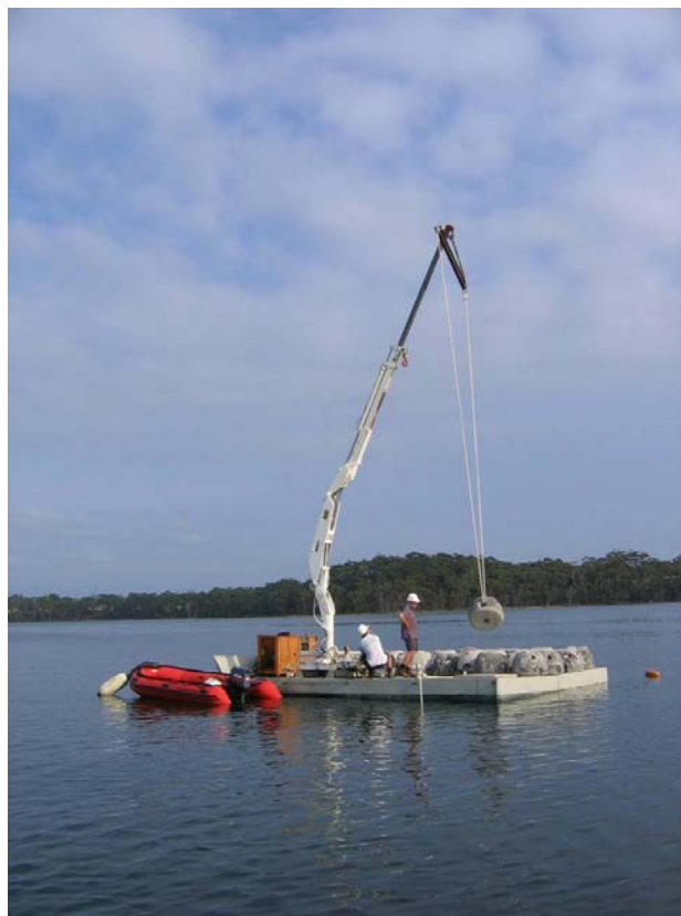
Figure 6 – Installation of Reef Balls by barge in St Georges Basin
