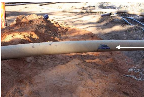
The pipe with the wipe mark, showing the point where the pipe is thought to have struck Mr Austin.
