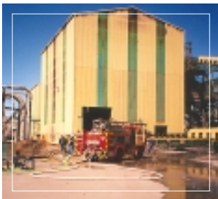
'Hot work' incident resulted in major damage to an operation's crushing plant
